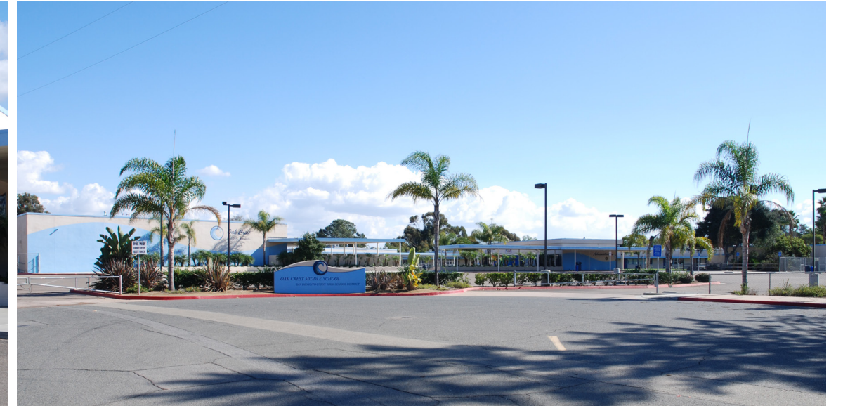
View of main entry into the campus. This cul-de-sac is very congested during the morning and afternoon periods.
