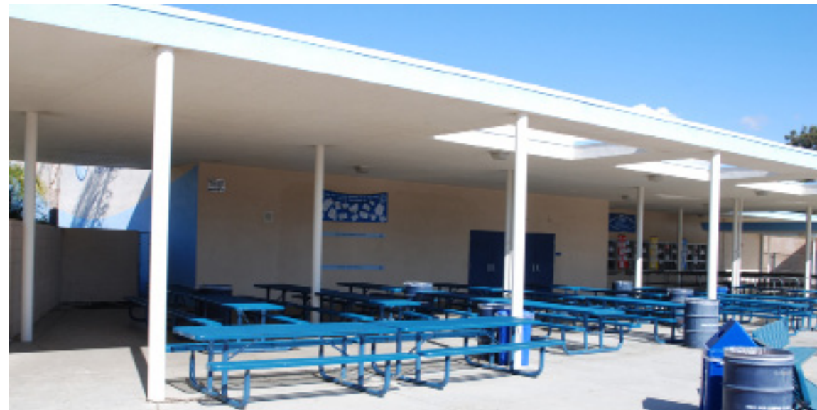
View of the lunch eating area multi-purpose building.
