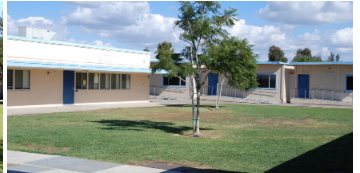
View of landscaped area. the low walkway canopies and portables classrooms to the east
