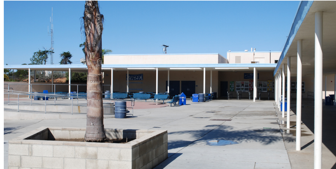
View of multi-purpose building from south of the plaza area.
