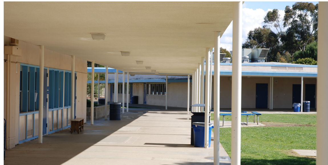
Typical view of walkway canopies throughout the campus. The walkways have low ceiling and gives a compressed linear environment on the campus
