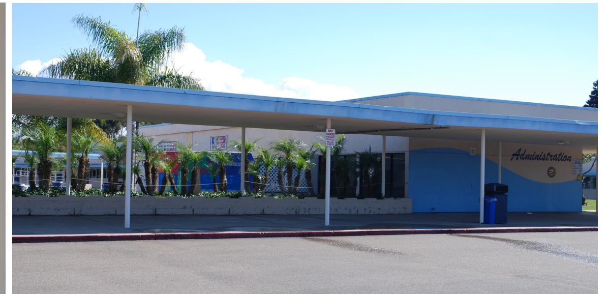
View of Administration Building from the parking area.
