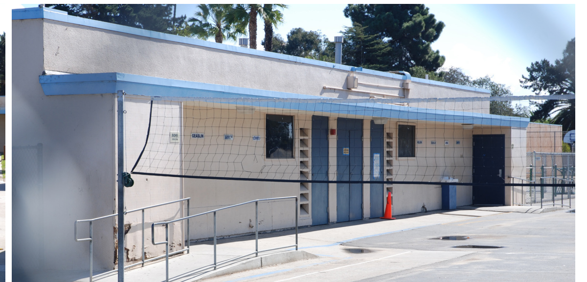
View of student locker building. This building has reached its useful life and needs replacement.
